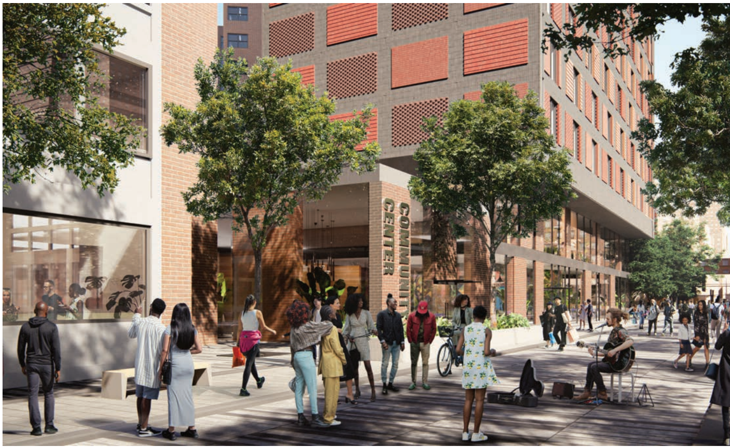
THIS RENDERING OF THE NEW BUILDINGS PROPOSED FOR THE ELLIOTT-CHELSEA HOUSE CAMPUS , hints at cultural activities and amenities on the lower floors, and a city-street atmosphere. Credit: NYCHA.
