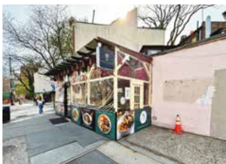
FATOUSHA RESTAURANT at the corner of Seventh Avenue South at Commerce Street has improper structures on the sidewalk as well as plastic sheathing and garish advertisements.
