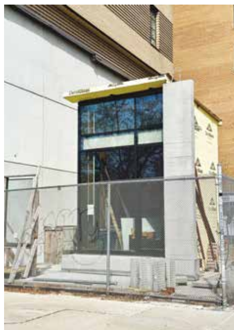
ERECTED IN 2023 , this temporary mock-up room for the residential building at 140 Jane Street is on an empty lot on the West Street corner, allowing testing for thermal and moisture performance of the materials assembly. It also gives us a preview of a part of the exterior appearance. This view is looking east from the Hudson River Park at West 12th Street. Credit: Brian J. Pape, AIA.
