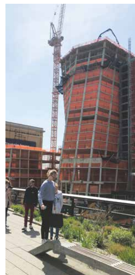
THIS 2021 VIEW OF ONE HIGH LINE is looking west from The High Line Park. It was stalled in a partially-complete state for many months when the developer went bankrupt. Credit: Brian J. Pape, AIA.
