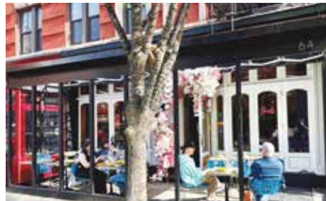
SVETA at 64 Carmine Street has improper structures on the sidewalk including an illegal roof.
