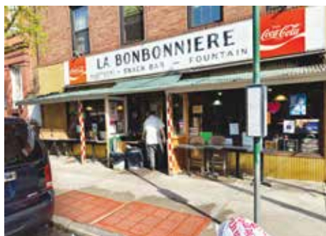
LA BONBONNIERE at 28 Eighth Avenue refuses to remove their improper structures on the sidewalk. The entire storefront has a makeshift roof with posts over the sidewalk where it doesn’t belong.
