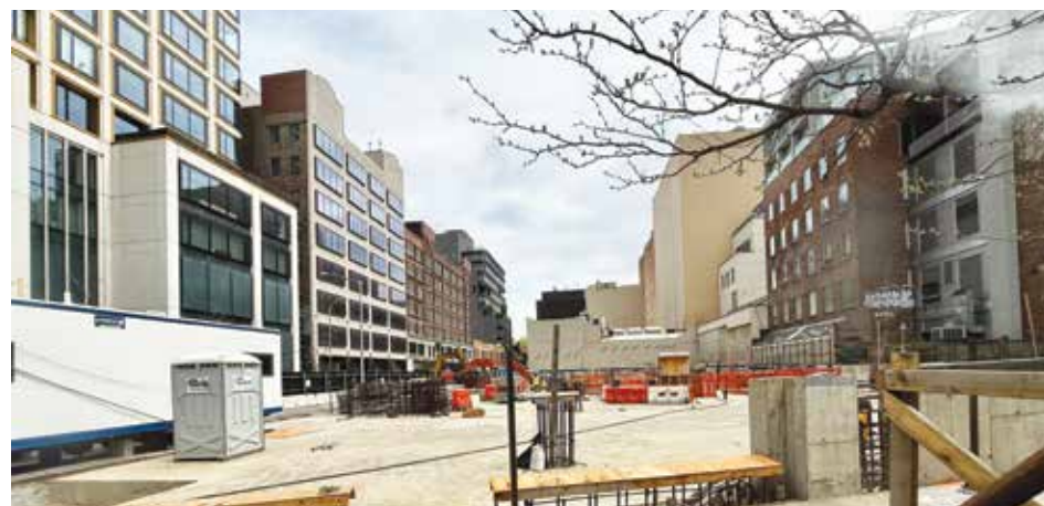
CONSTRUCTION HAS RESUMED at 550 West 21st Street, according to YIMBY. Above-grade work has continued recently, after construction was stopped at the site in 2023. Grade-level floors have been in place between the foundation walls to brace the perimeter construction poured. This view is looking east from West Street. Credit: Brian J. Pape, AIA.
