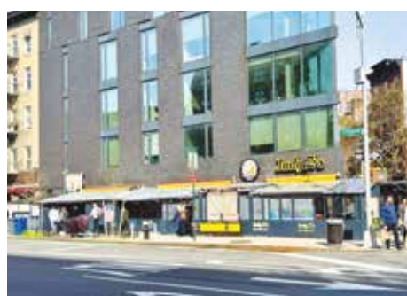
JUDY Z'S at the corner of Seventh Avenue South and Carmine Street refuses to remove the improper structures on the sidewalk many months after they were required to take them down. Note the shed beyond the corner where it doesn’t belong. A huge business bus seems permanently parked on Carmine Street.
