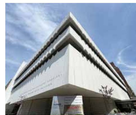
A NEWLY EQUIPPED HOSPITAL is opening on the site of the former St. Vincent's Medical Center in Greenwich Village. Photo credit: Buck Ennis.
