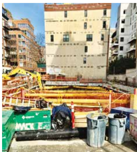
FOUNDATION WORK HAS PICKED UP at 140 Jane Street, according to YIMBY. Below-grade work has gradually resumed recently, after excavation and pilings were stopped at the site in 2024. Banks of yellow cylindrical struts have been in place between the foundation walls to brace the perimeter construction. Note the backhoe digging out between the struts, still in place despite concrete foundation walls poured in 2023. This view is looking east from West Street. Credit: Brian J. Pape, AIA.
