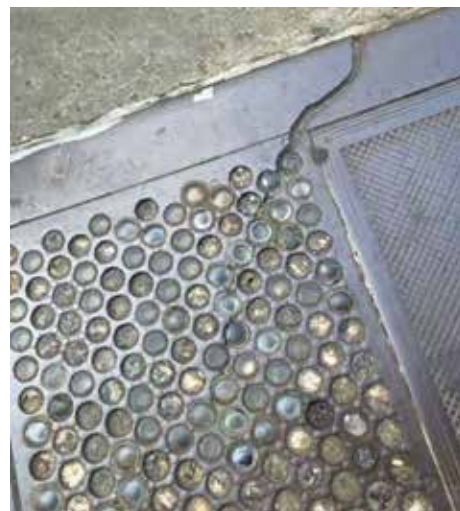
THIS CLOSE-UP OF THE 54 GREENE STREET vault lights shows broken glass beads and cracked metal frames, allowing water to penetrate into the basement vaults. Credit: Beyhan Karahan & Associates.
