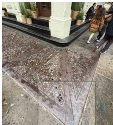
THESE SIDEWALK VAULT LIGHTS are at 54 Greene Street at the Broome Street corner. The circles are glass beads that allow daylight into the basement vaults. Credit: Beyhan Karahan & Associates.
