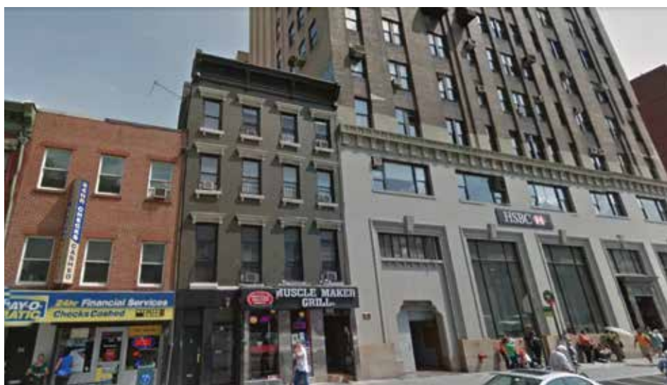
PRIOR TO HURRICANE SANDY , 92 Eighth Avenue, center, had been a four-story, mixed-use walk-up built around 1910. Credit: Apartments.com.
