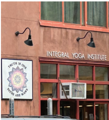
INTEGRAL YOGA INSTITUTE ON WEST 13TH STREET is being renovated. Photos: Roger Paradiso.
