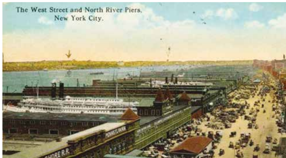
THE WEST STREET AND NORTH RIVER PIERS, New York City. Credit: New York Public Library.
