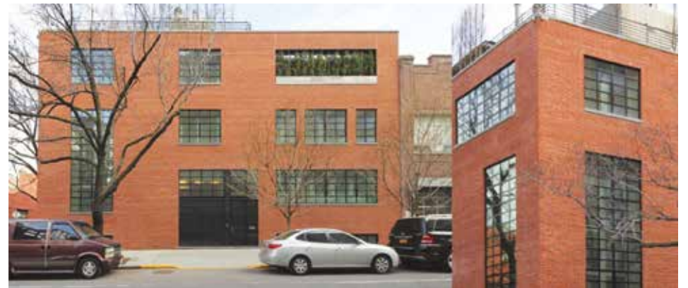
THIS QUIET BRICK BUILDING is a former warehouse that was repurposed for an art collector. Generous, landscaped roof terraces add to the ambiance of the single-family residence at Washington and Jane streets. Credit: Leroy Street Studio.
